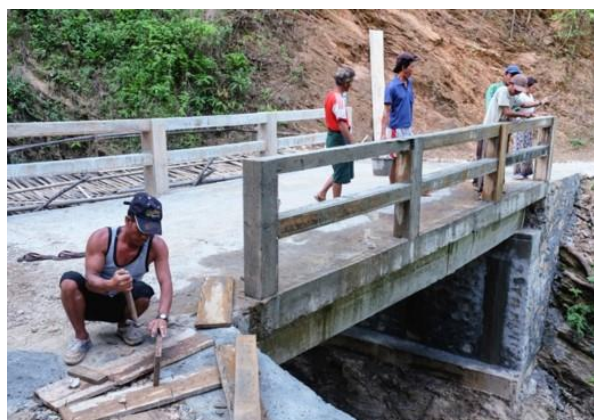
Community in charge of bridge construction
