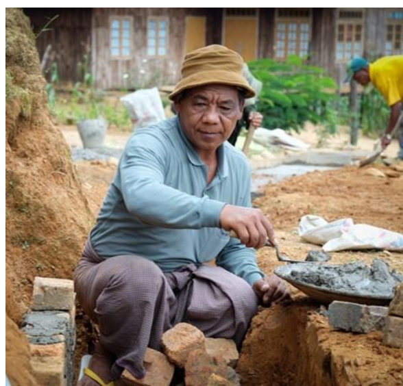
Construction of drainage
