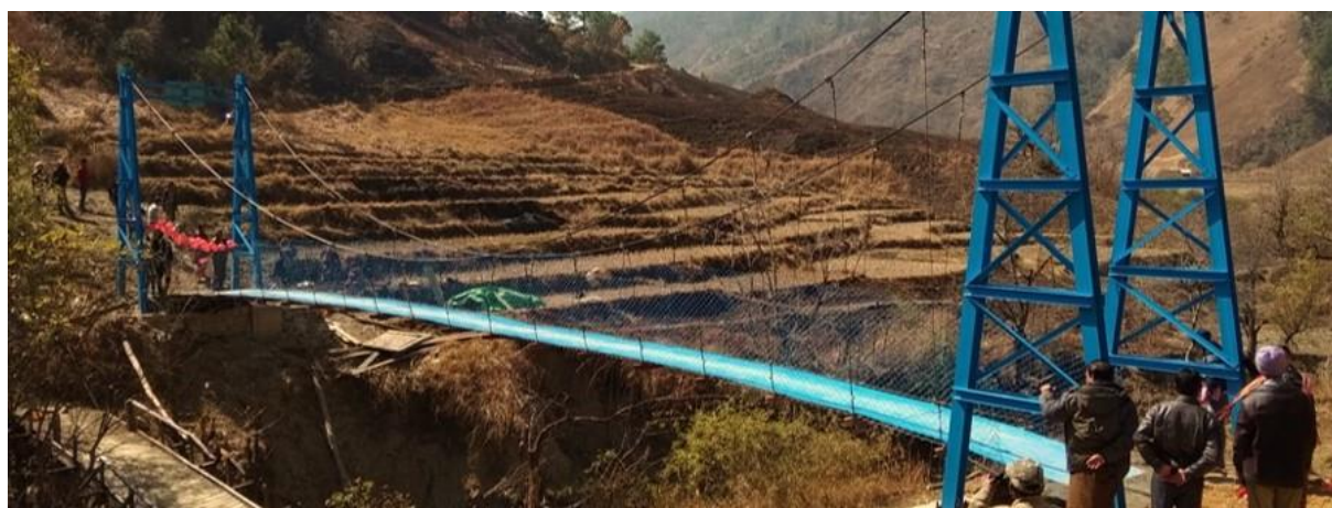
Suspension bridge to support connectivity
